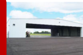
Hangar LFZ (Code B)
